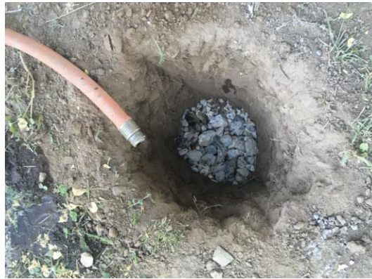
Figure 7: Percolation Test Hole
